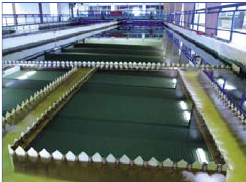
Štítary, water preparing plant
